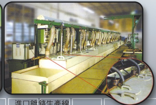
進口鍍鉻生產線 CHROME PLATING LINE
